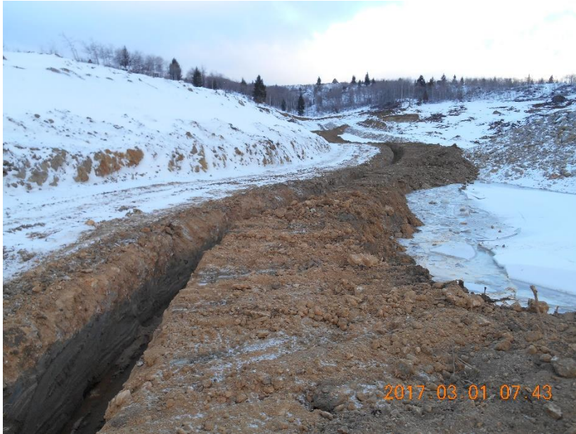
PHOTO 3 – Well DH15-12, Piezometer Cabling Trench. Looking West. March 1, 2017.
