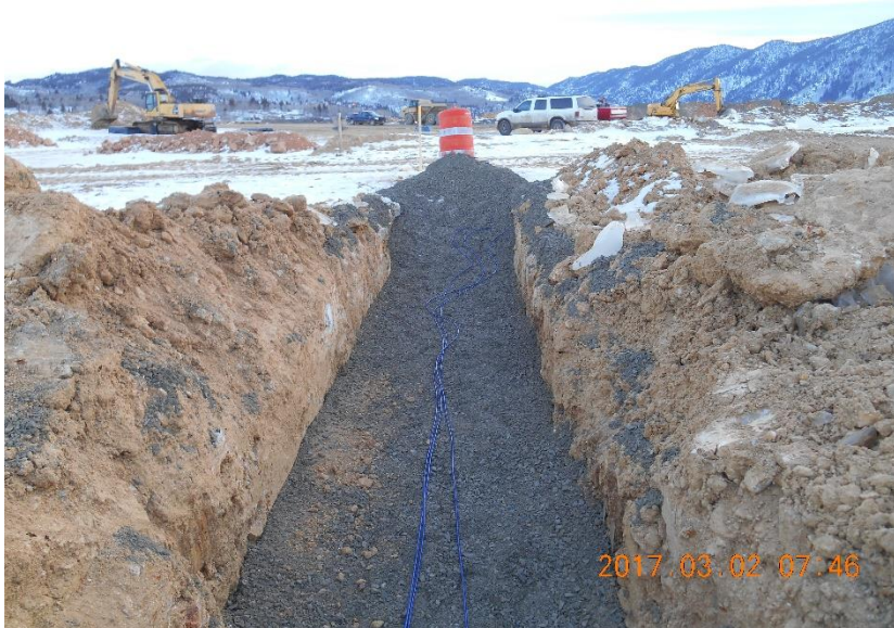
PHOTO 4 - Well DH15-12, Piezometer Cabling Trench. Looking North East. March 2, 2017.
