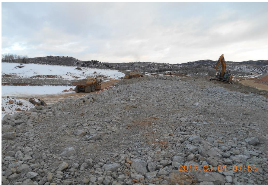
PHOTO 2 - WED – Placement of UA Cap Rock, Station 27+00, Looking North. March 1, 2017.
