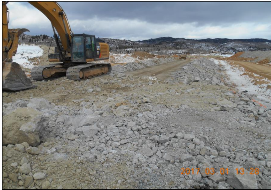
PHOTO 1 – West Embankment Drain (WED) - Station 27+00, Placement of UA Protective Cap Rock. Looking North. March 1, 2017
